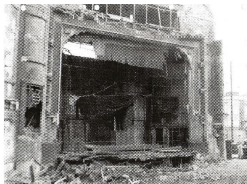
The remains of the Troc-ette during demolition
